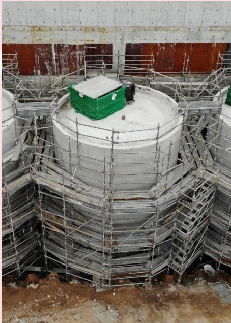
Construction of Sludge Holding Tanks 污泥貯存缸工程
