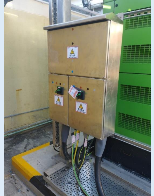
Installation of Distribution Board 配電箱安裝工程
